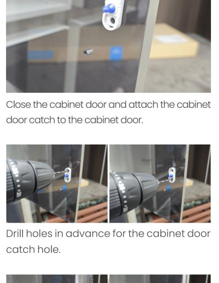
Fasten the cabinet door catch to the decorative cover, and the cabinet door catch installation is completed.
